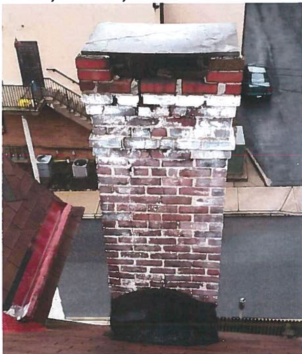
Chimney is severely deteriorated and should be removed
