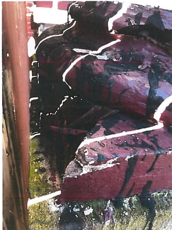
Columns on North Side deteriorated and rotted
