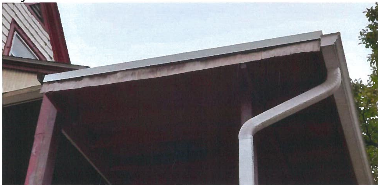
Siding deteriorated
